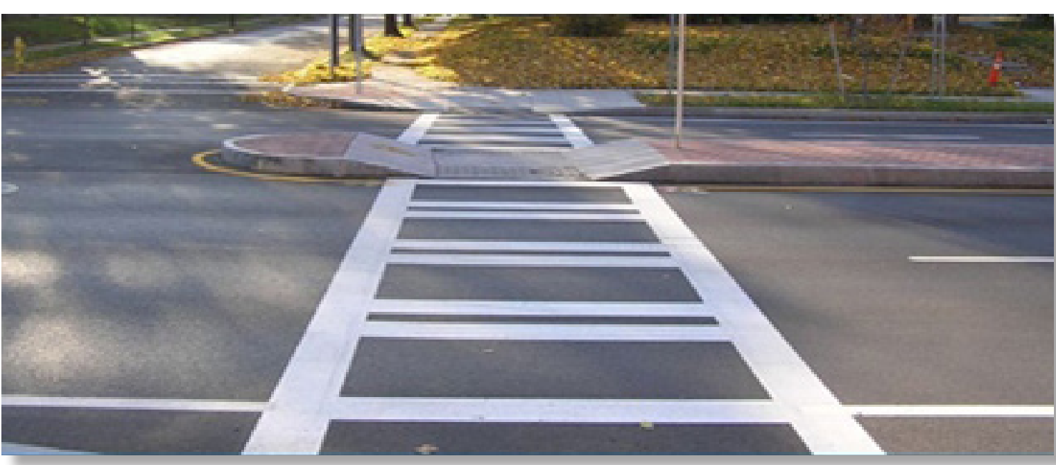
Figure B: Raised median with crosswalk cut-through (aka refuge island); Photo source: highways.dot.gov
